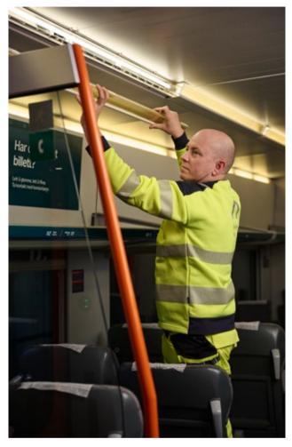
Hans Ingar Fossen dismantling an old light tube containing mercury. They are to be replaced with new led lights.
