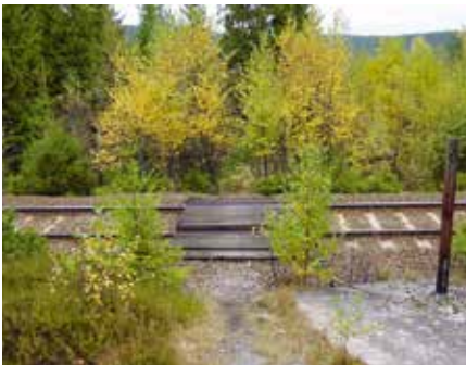
Usikret planovergang/Ungated level crossing
